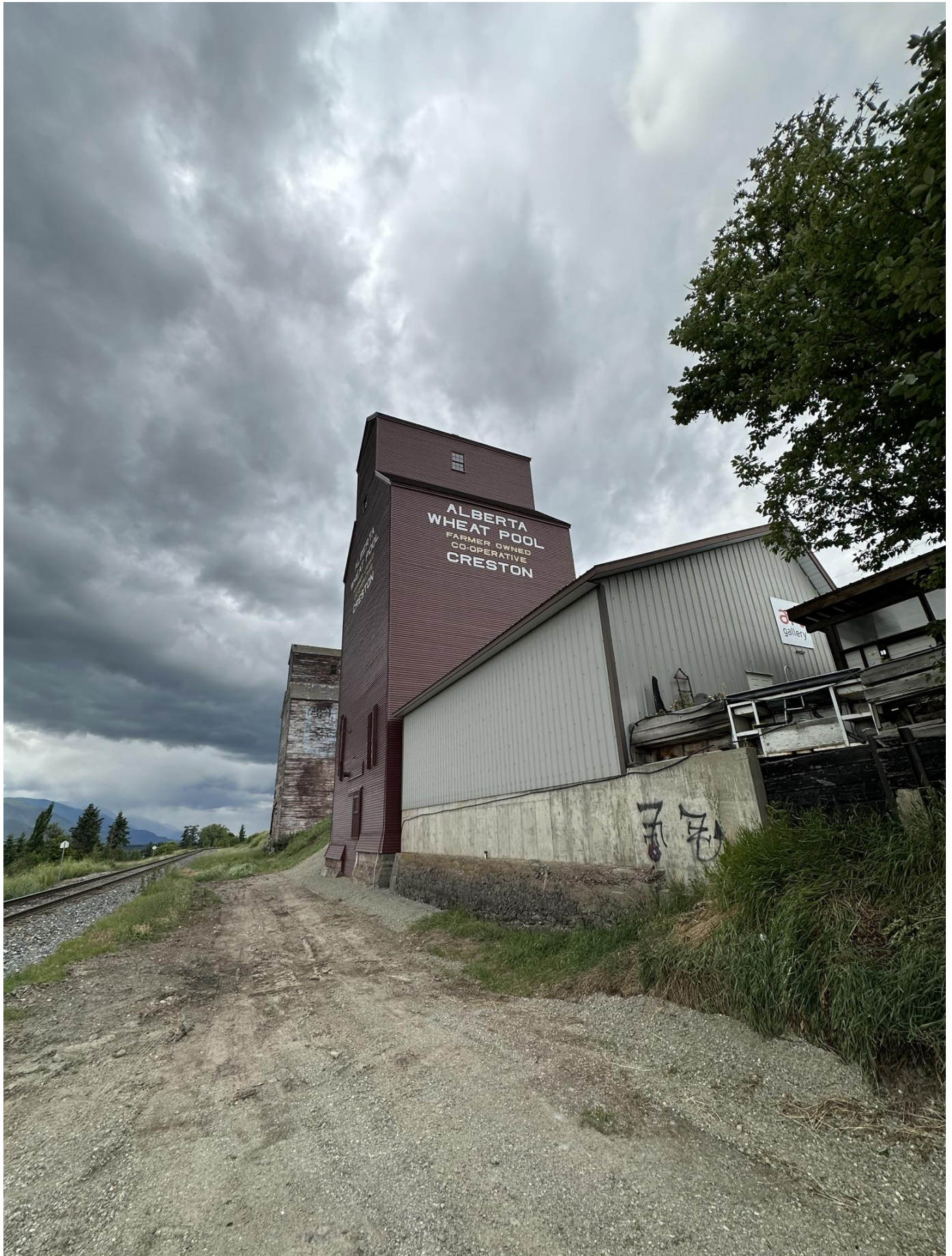
Figure 7: West property line, facing North
