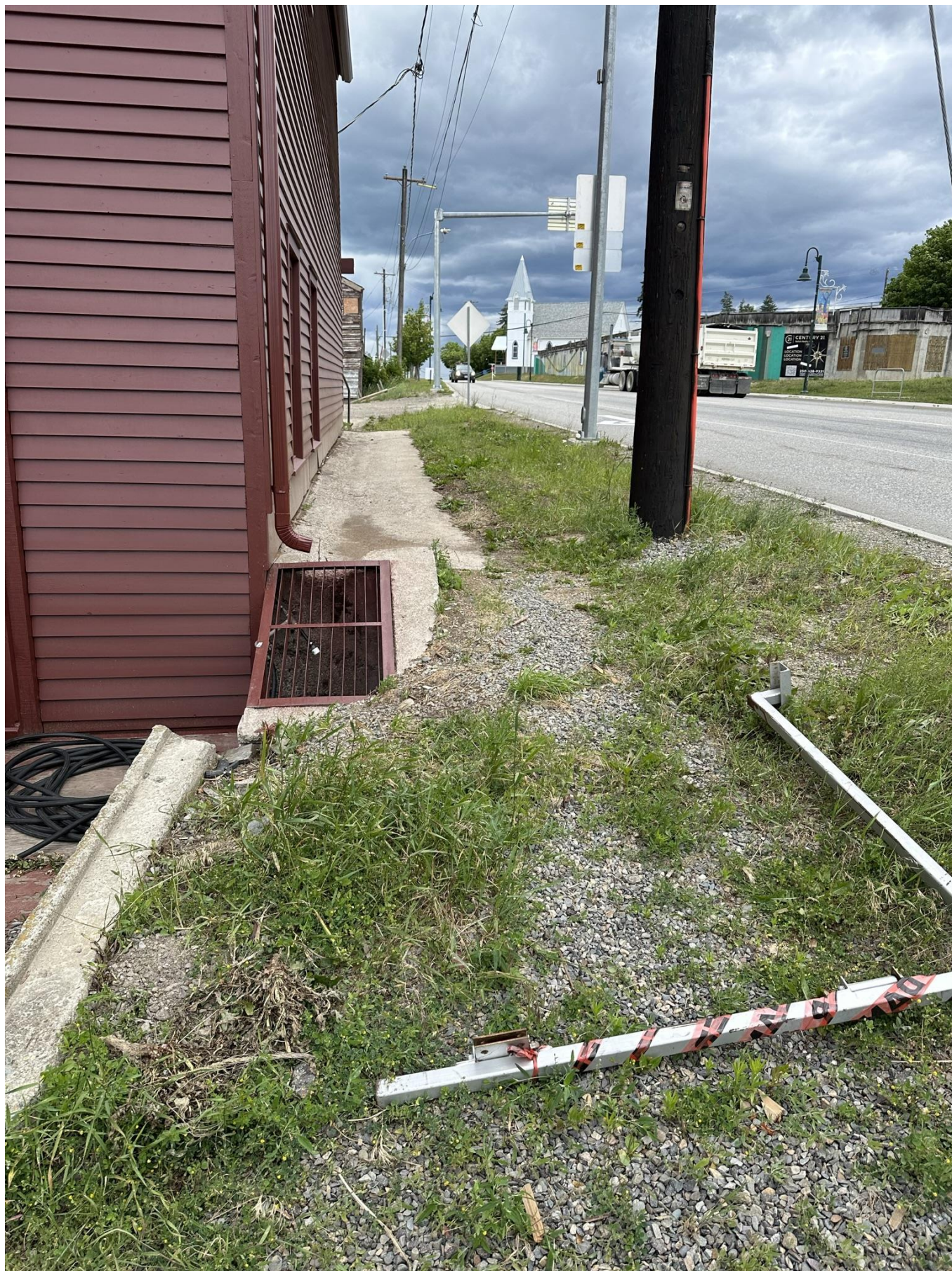
Figure 5: Sidewalk area – south facing north
