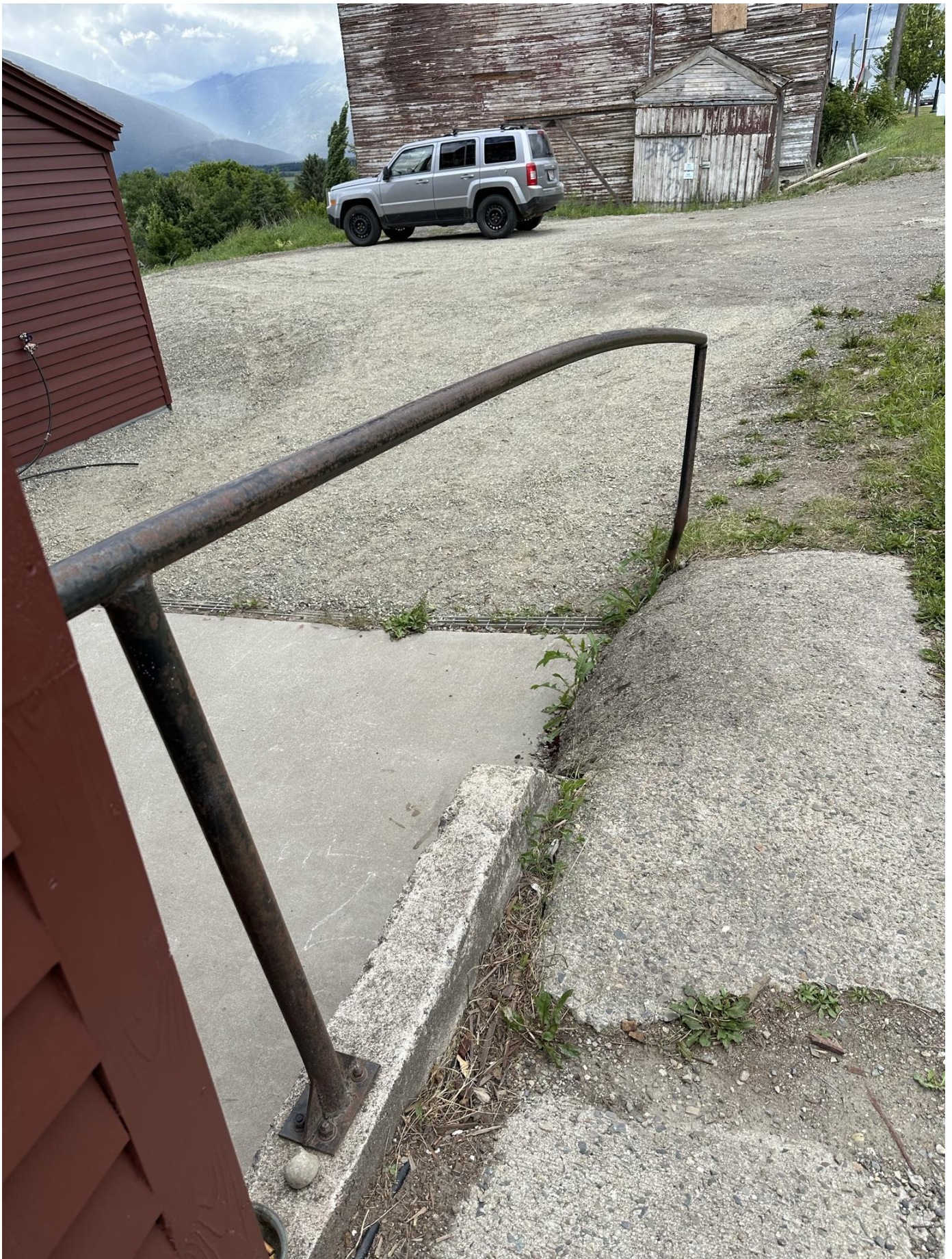
Figure 4: Sidewalk area – north entrance
