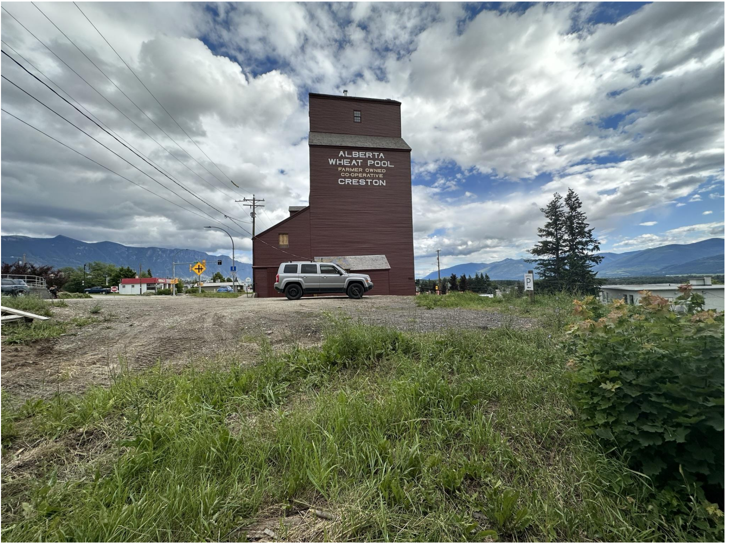
Figure 1: North edge of parking lot, facing South.
